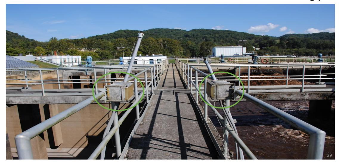
Aeration Basin. Ammonia is removed here. Has original gear boxes and parts no longer available.
