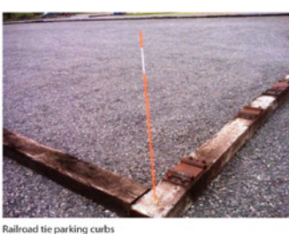
Railroad tie parking curbs
