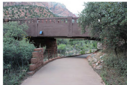
Trail passing under rail line along the Pa'Rus trail in Arizona.
