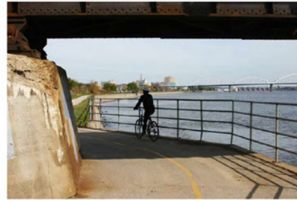
Mississippi River Trail crosses under an active rail line in Rock Island, Illinois.
